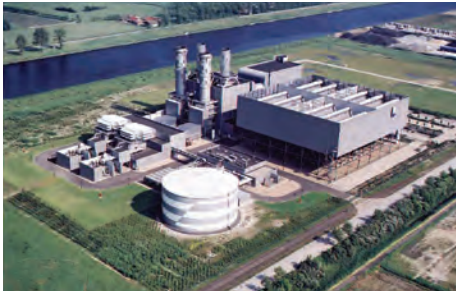
Bruges, Belgium — ACC for 460 MW Combined Cycle Power Plant.
