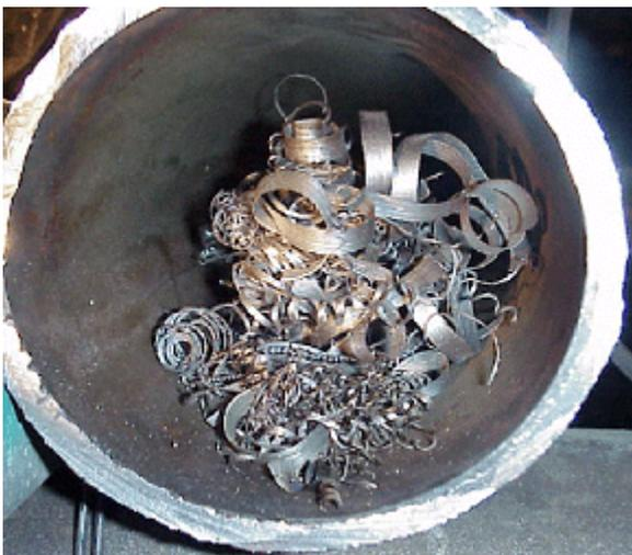
**Figure 1. Metal Shavings found in piping following the Fitting Process**
