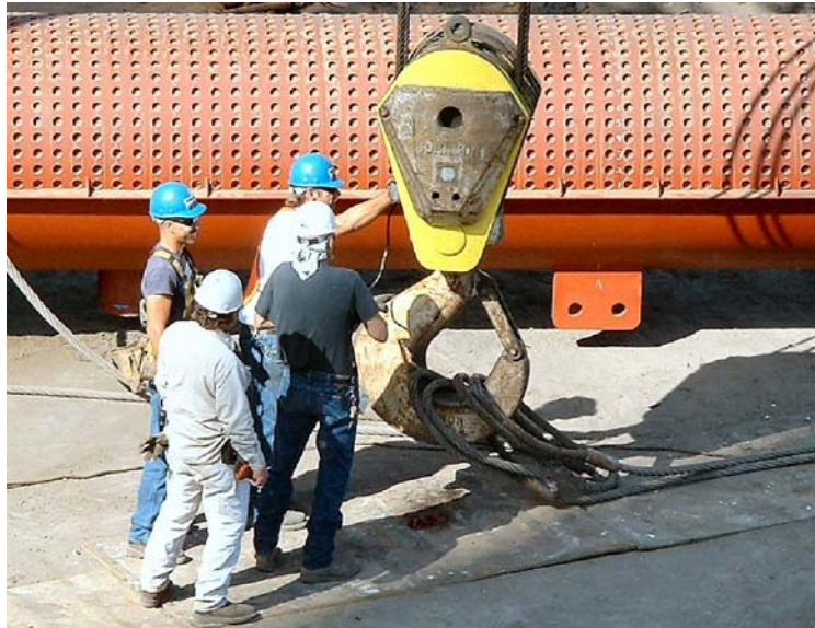
Fig. 7 Mud Drum Erection
